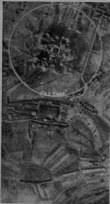
Marshalling Yards ( St. Wendel )
